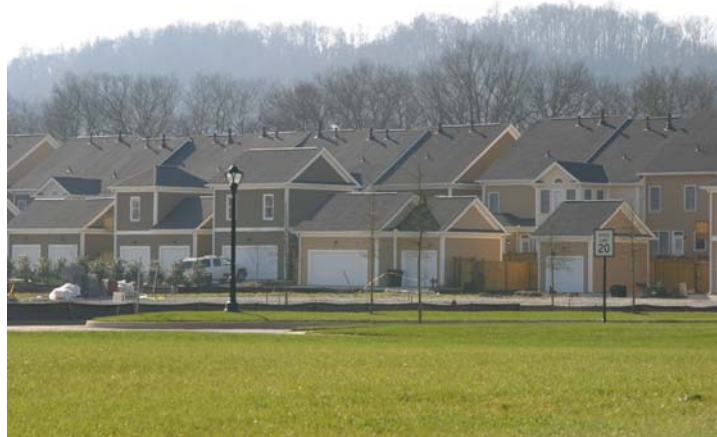
Figure 2-4: This image shows detached garages (facing onto an alley prior to the completion of the homes on the opposing street) with some two-story garages that accommodate an accessory dwelling unit.
