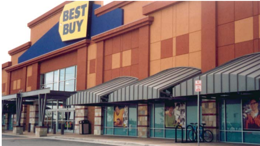
Figure 3-25: This large retail center utilized several different design features to articulate the individual facade and customer entrances.
