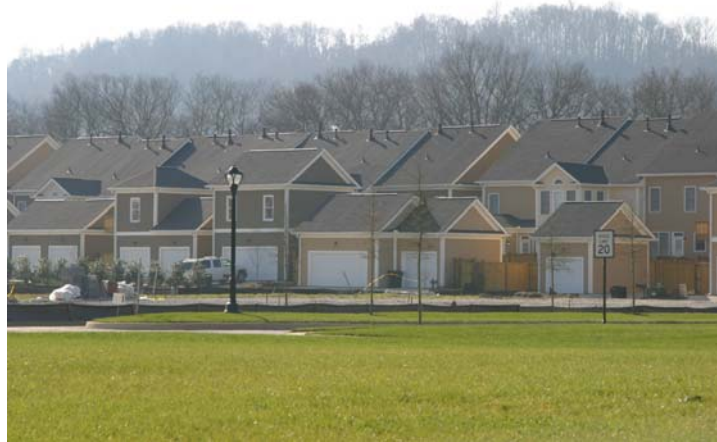
Figure 2-4: This image shows detached garages (facing onto an alley prior to the completion of the homes on the opposing street) with some two-story garages that accommodate an accessory dwelling unit.
